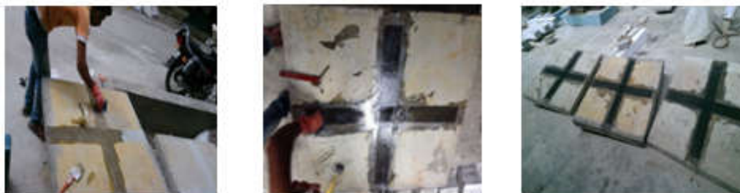
Fig.4. -Application of BFRP Sheets
