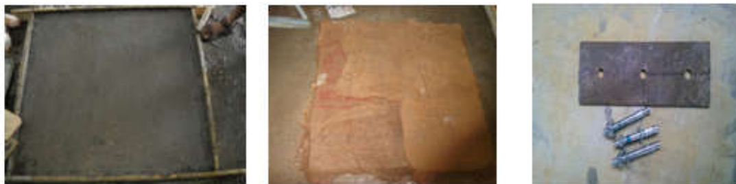
Fig.3. Compacted concrete, Curing of slab using gunny bags, and anchor bolts and plate
