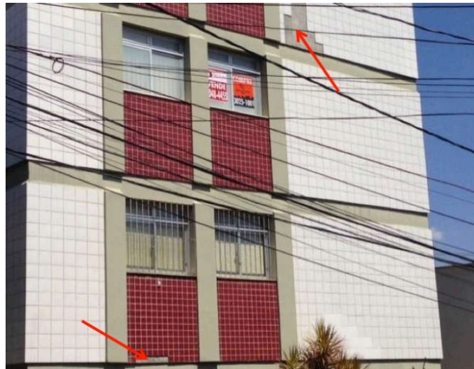
Figure 1. Detachment of ceramic coating on external facades
