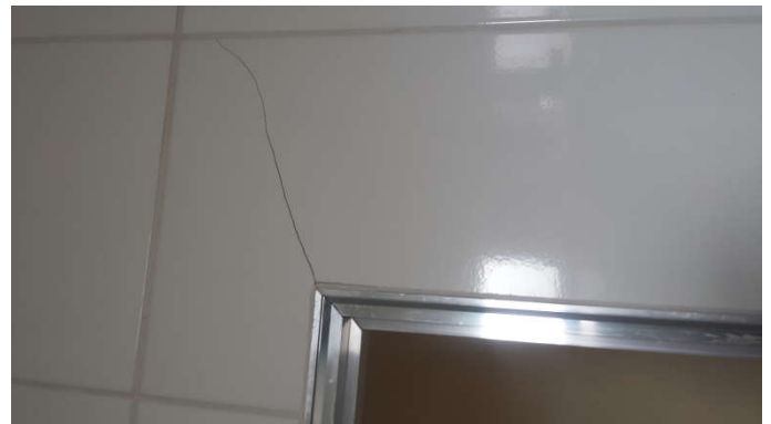
Figure 10. Crack observed in an inner door of the building
