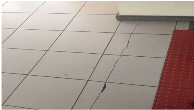
Figure 3. Broken due to excessive deformability
