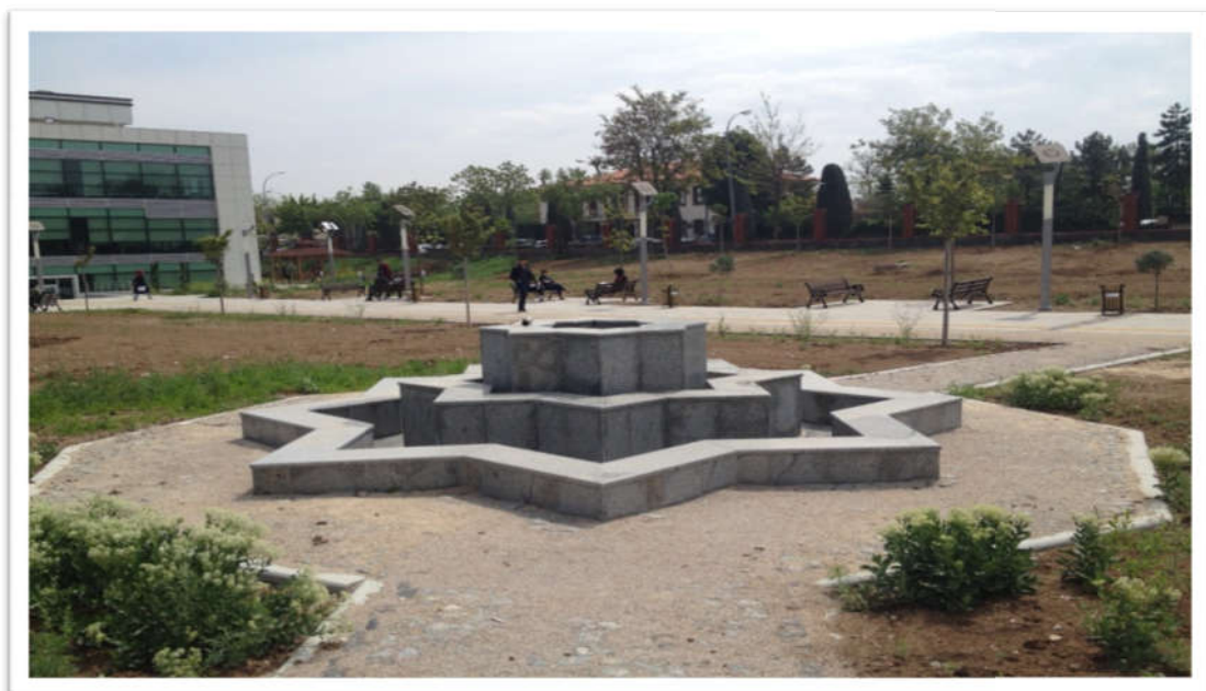
Figure 7. The cascaded fountain pool in July 15 campus
