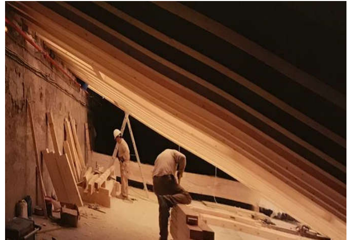
Figure 6. wood restoration works
