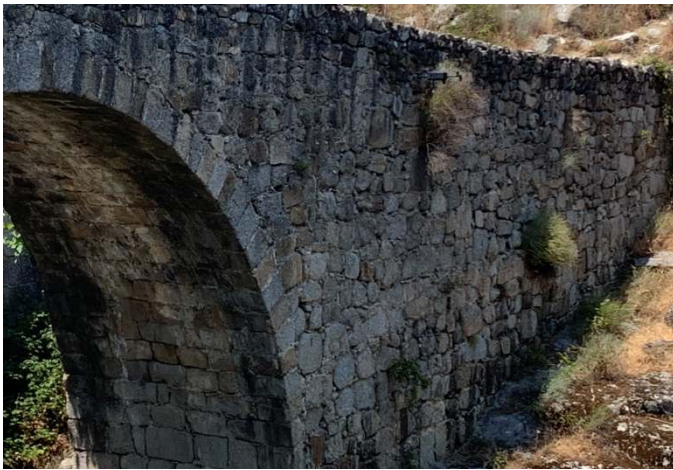
Fig. 3. Drone approaching to the medieval Bridge for its inspection (photograph taken by the autor)
