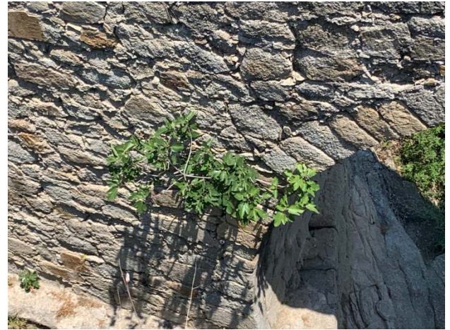
Fig. 8: Image captured with the quadcopterdrone, where you can see vegetation (a fig tree) rooted in the joints of the masonry (photograph by the author)
