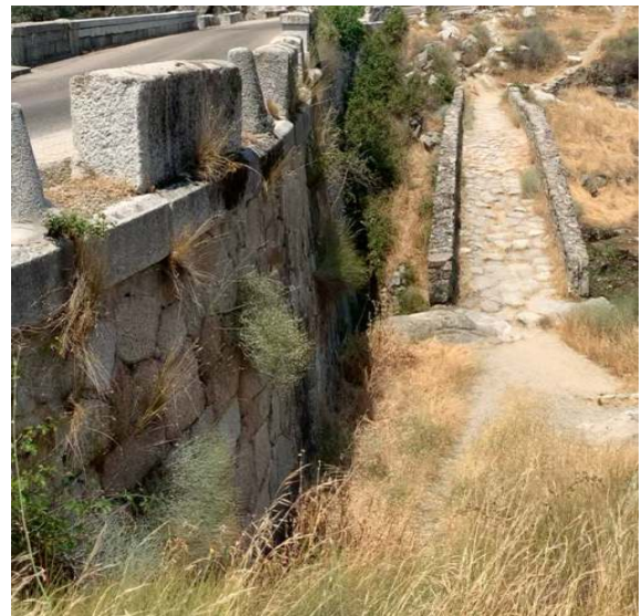
Fig. 2: Roadway over the medieval bridge (right) and traffic road over the nineteenth-century bridge (left). It gives an idea about the separation between the two bridges (photograph taken by the author)
