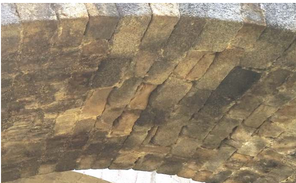
Fig. 7: Image captured with the quadcopterdr one in the intrados of the upper part of the vault, where in addition to the previous injuries Fig. 5 y Fig. 6 we observed vesiculation of ashlars (author's photograph)
