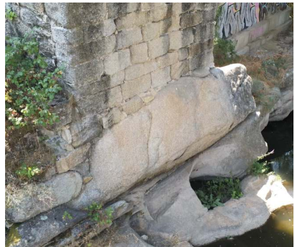
Fig. 4. Photograph taken with the drone, where the found ations of the eastern abutment of the Medieval Bridge can be seen (photograph taken by the autor)
