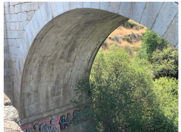
Fig. 9: Image captured with the quadcopterdr one in the intrados of the vault of the new bridge, with lesions identical to those of the medieval bridge being observed: efflorescences or dark crusts (photograph by the author)
