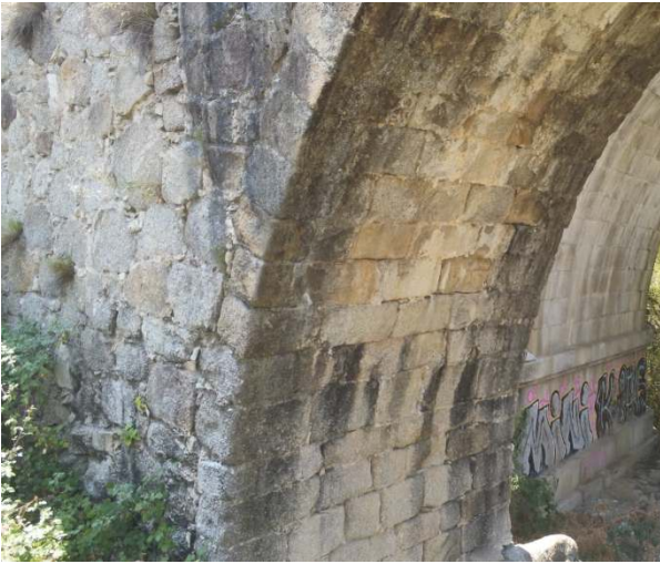
Fig. 6: Image captured with the quadcopterdr one at the eastern start of the vault, where various lesions can be observed, such as efflorescence or dark crusts (photograph by the author)
