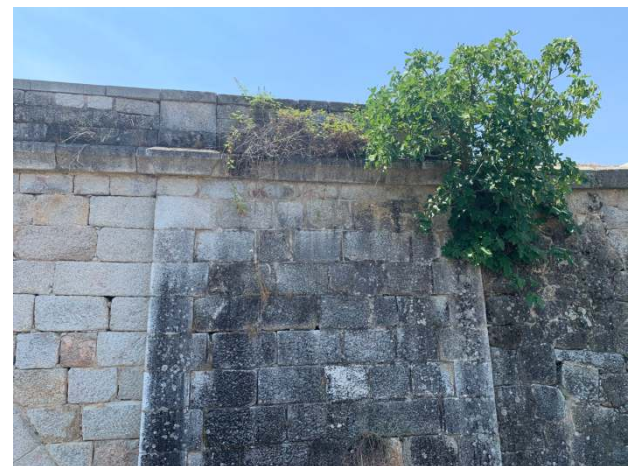
Fig. 10: Image captured with the quadcopterdrone, where a detail of the west abutment can be seen, with root edge vegetation, black crusts and run off watermarks (photograph by the author).
