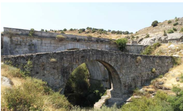
Fig. 1: Photograph taken with the drone used in the inspection, where we can see the Grajal Medieval Bridge, north elevation, with the nineteenth-century bridge behind it (photograph by the author)
