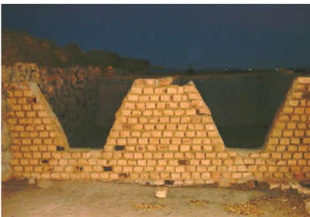
Figure 1. A kind of silo which used for urea treatment (Iran)
