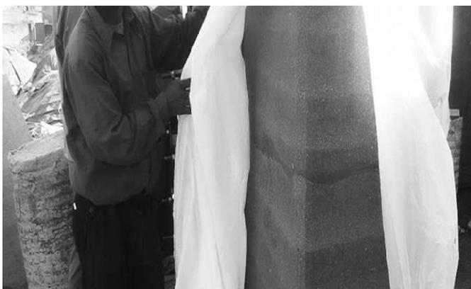
Figure 17. Rammed Earth used in the Mato Ghar
