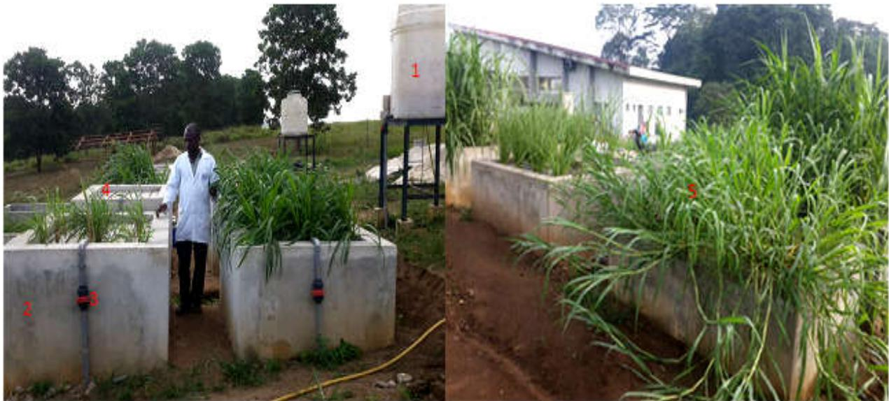
Fig. 1. View of the pilot-scale constructed wetlands (CWs): feeding tank (1), bed (2), water supply valve (3), irrigation device (4), and plants growing on the beds (5).
