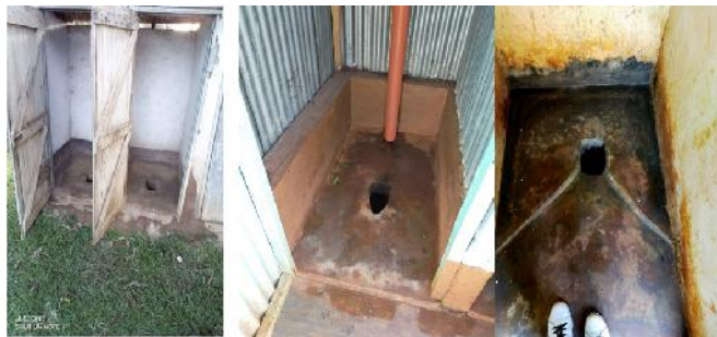
Health facility toilet codes M002, R001 and N001
