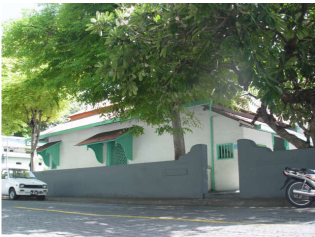
Fig 2. General View of Dharumavantha Rasgefaanu Mosque before conservation
