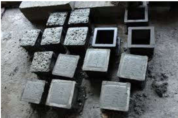
Figure 2. Casting of cubes
