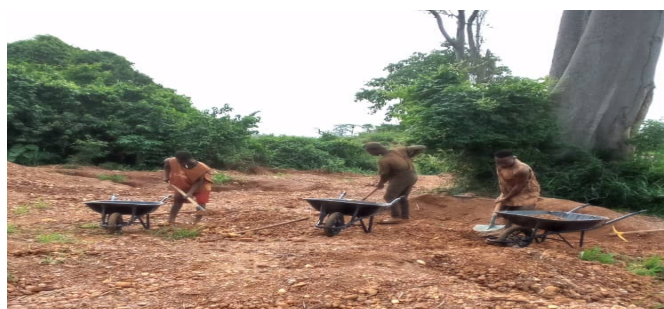
Figure 6. Closing the pits with aggregates
