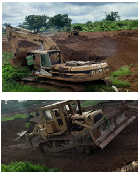
Figure 3. Machines carrying out backfilling
