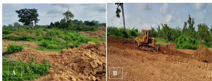
Figure 7. Before and during backfilling
