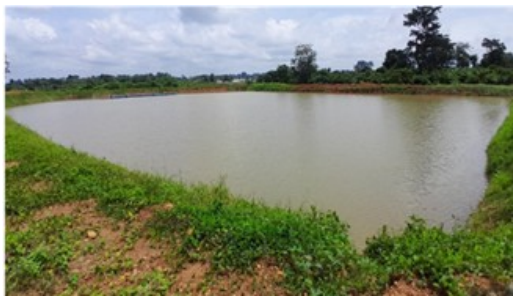
Figure 10. Development of a fish pond (start and end of work)
