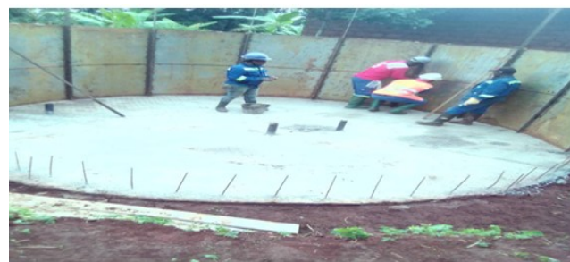
Photo 5. Reservoir under construction in Bangang
