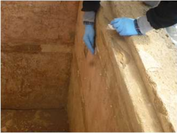
Figure 4. Sampling procedure performed on stone surface of painted walls of the tomb n. 8 using nitrocellulose membrane. The surface of wall is very faded due to biological and chemical deterioration
